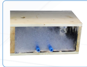
Cutaway model of a disinfectant foam application / pressing the foam into an underfloor structure after water damage
