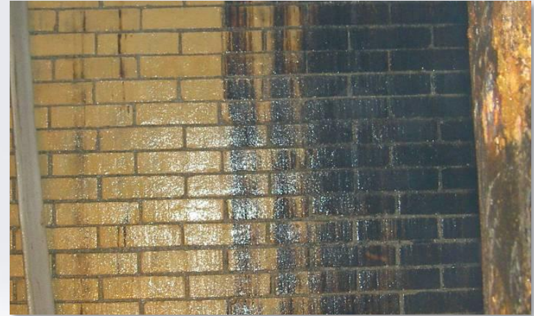
Left: cleaned with Clean TW- right: uncleaned
